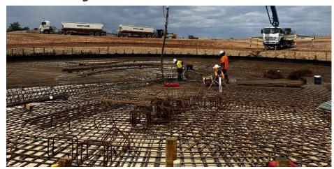
NOVA NACAP entrusted Bear Claw with the Civil and Concrete contract components to build two 4,000,000 litre "cut'n'cover" bulk fuel tanks and support infrastructure. This included pump houses, fill stands, utilities, site improvements, heavy duty pavements and other works necessary to provide a complete facility at the RAAF Base in Tindal.
